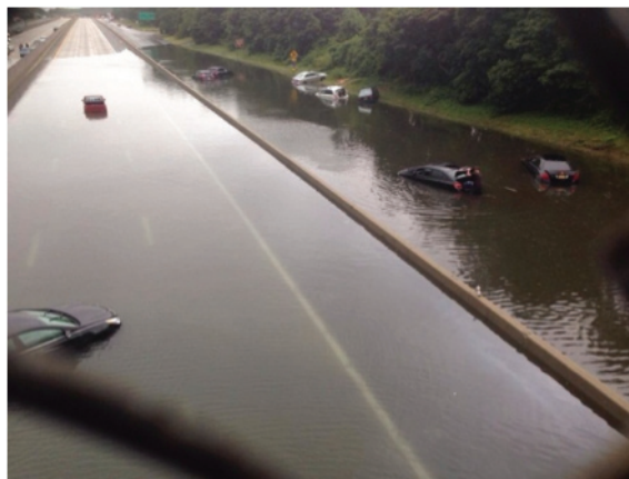
Islip, NY. Courtesy of the Islip Fire Department.
