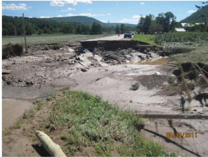
Flood of August 2011, State Route 30 road washout caused by Schoharie Creek at Breakabeen, New York. Photo by Joseph Griffin, courtesy of New York State Department of Transportation (USGS 2014).
